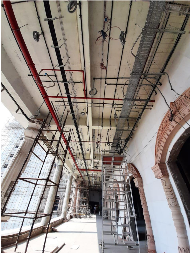
CEILING WIRING WORK- NT WING
