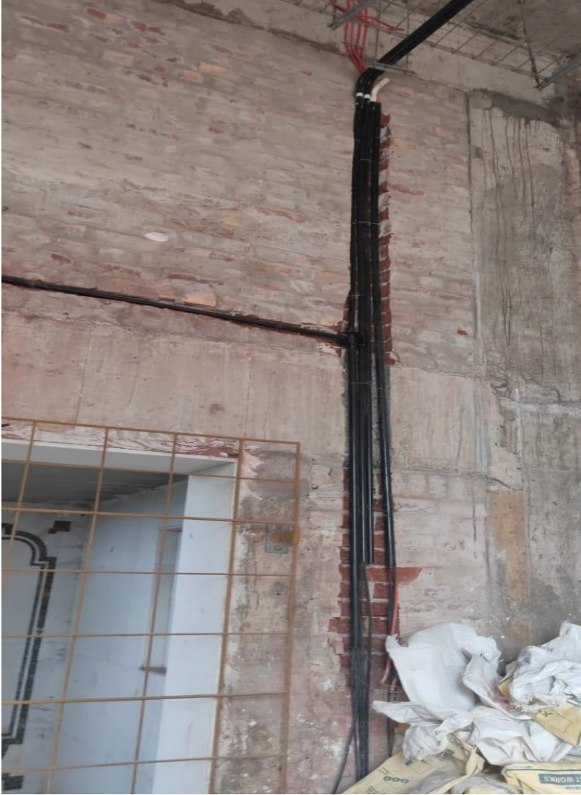
WALL CONDUIT FOR READER-M3 FLOOR
