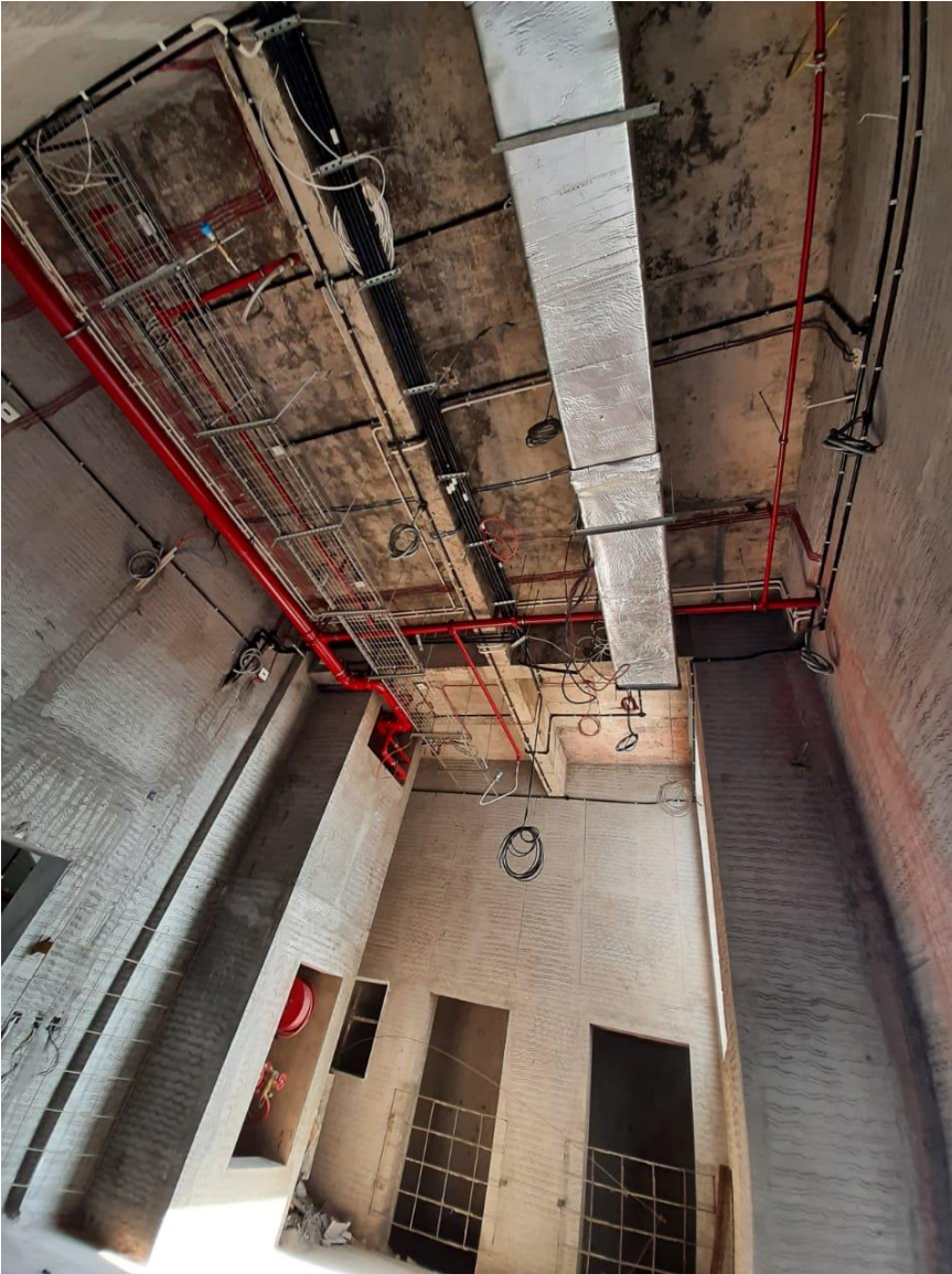
CABLE TRAY WORK- TEMPLE FLOOR NT WING
