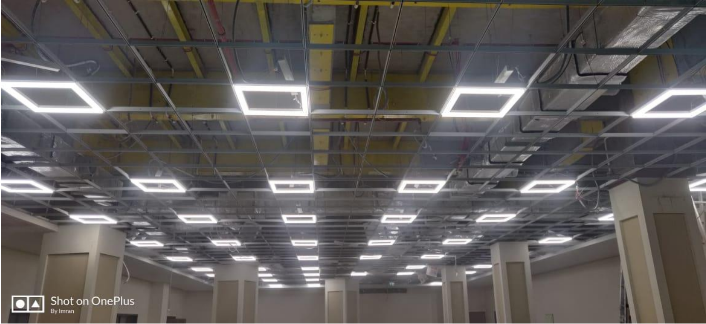
FESTIVAL ROOM-SLAB STRENGTHING DONE AND FINISHING IN PROGRESS
