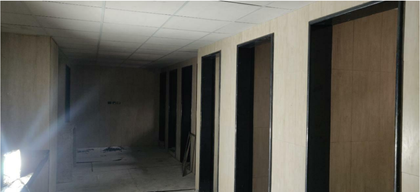
TOILET A-CEILING FINISHING IN PROGRESS
