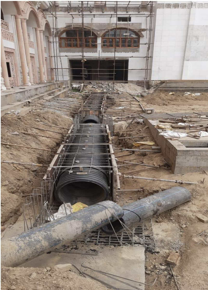
STROM WATER LINE- NORTH EAST SIDE
