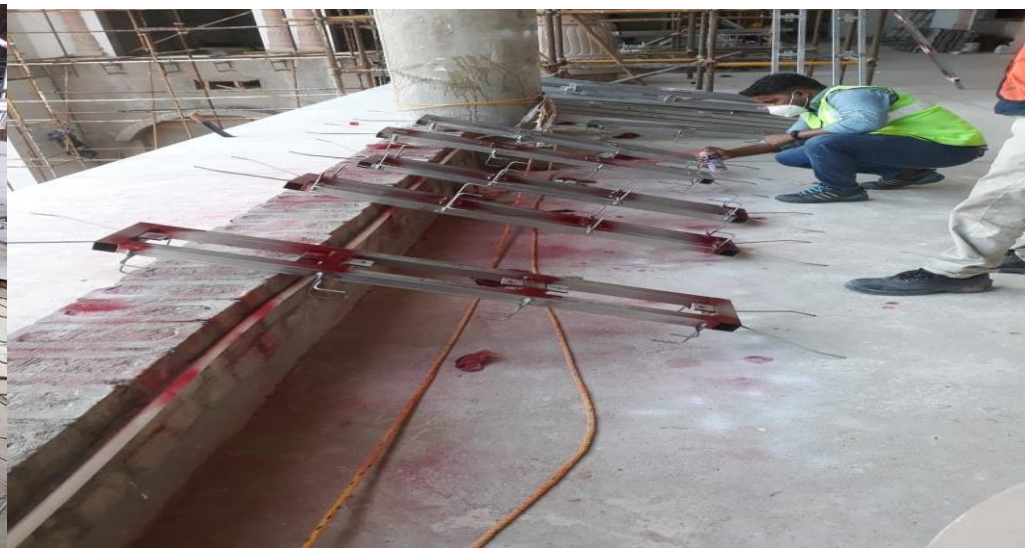
DYE PENETRATION TEST
