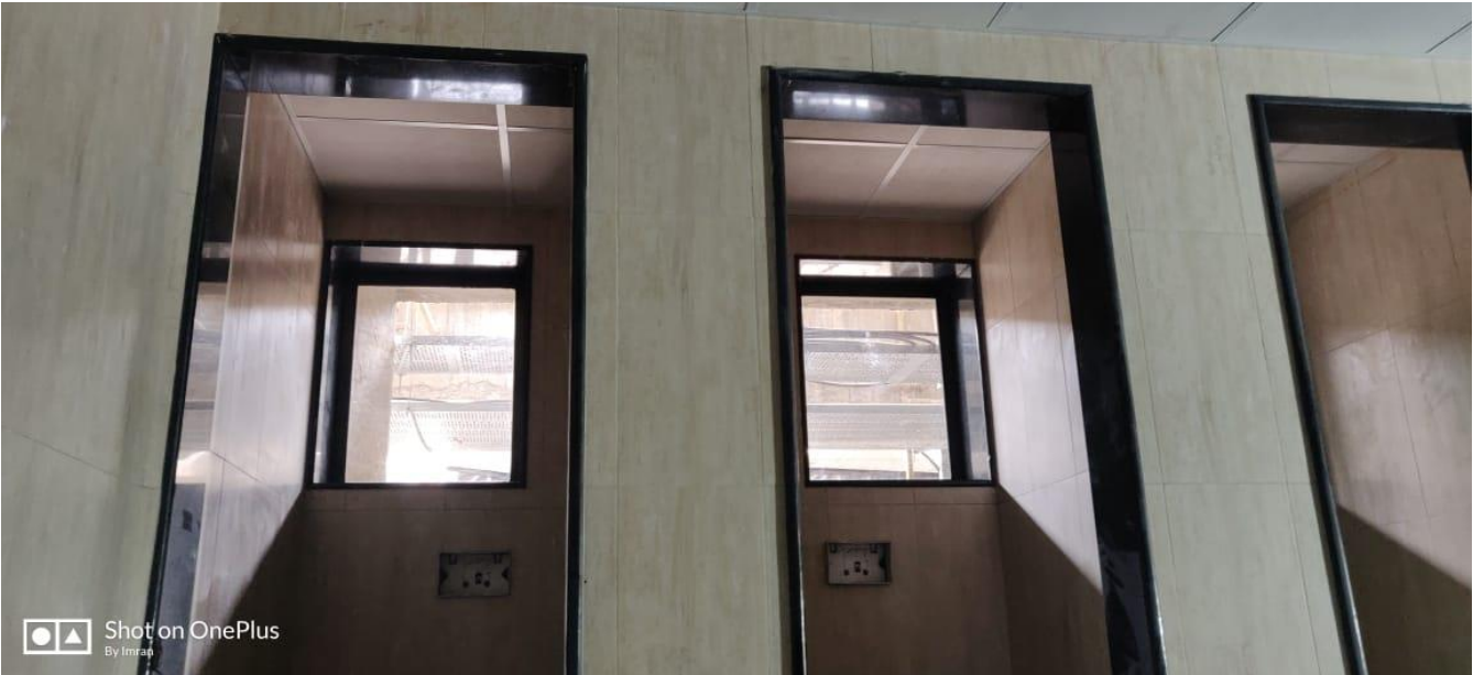
TOILET A-WINDOW FIXING IN PROGRESS
