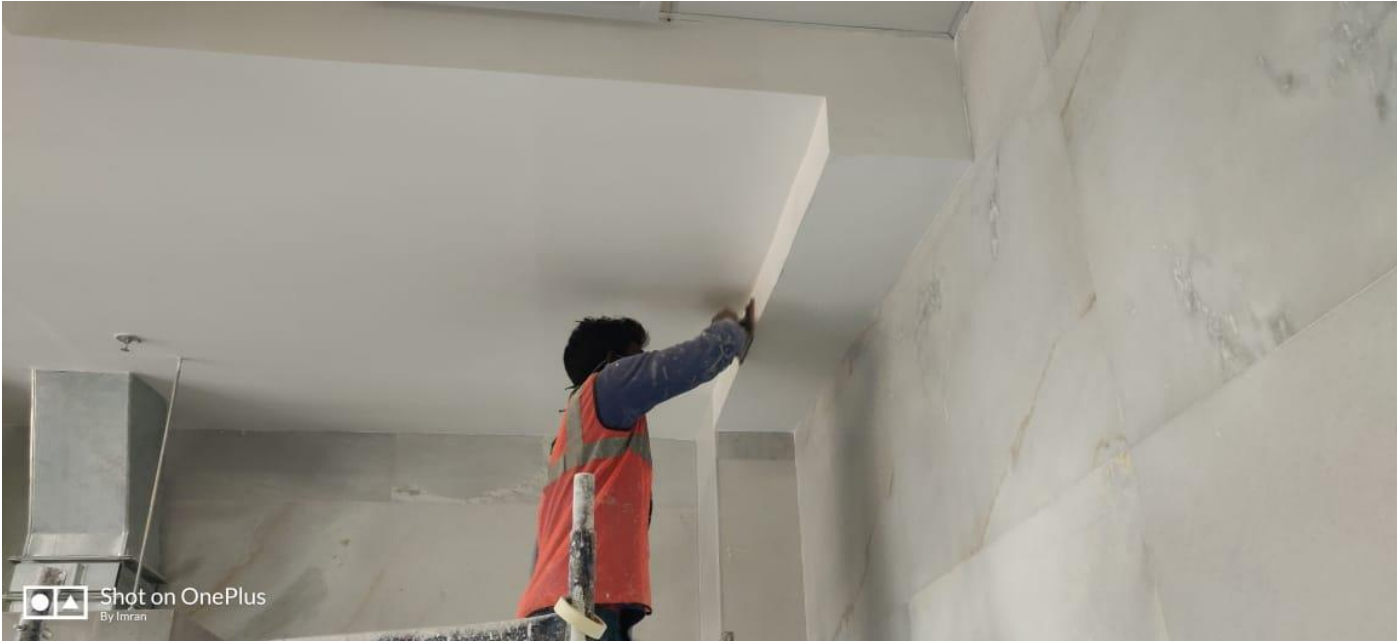
FESTIVAL KITCHEN-SNAG RECTIFICATION IN PROGRESS
